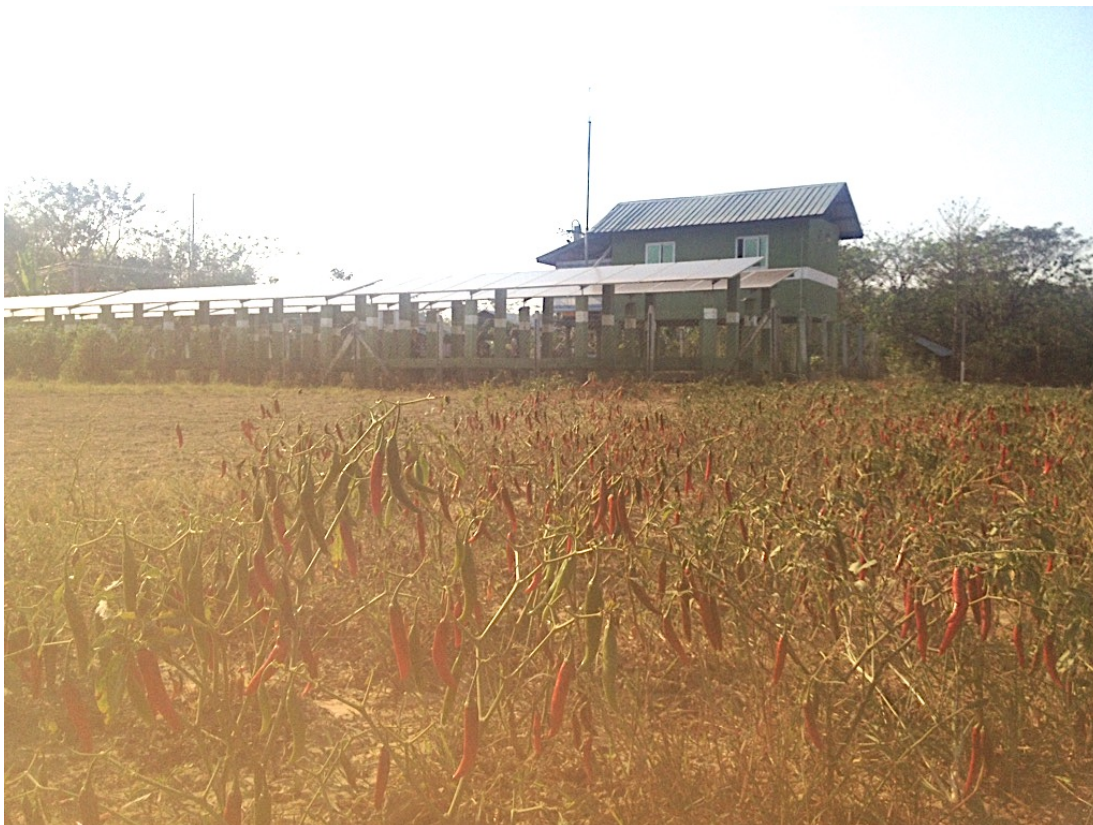
Figure 11 NEP-project solar plant
