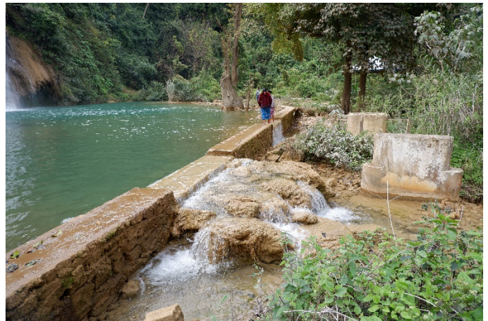
Figure 14 Water basin for a mini-hydro powerplant
